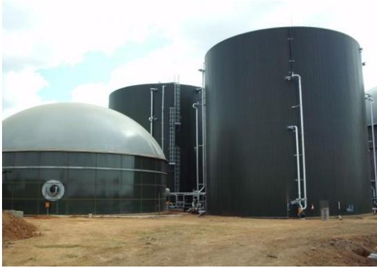
*Figure 3 Commercial anaerobic digester using cow manure and industrial waste, Source: Bio2Watt Bronkhorstspuit plant South Africa.*
