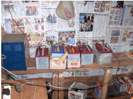
*Figure 2 Battery charging station using old car batteries at the Tungu Kabiri mini grid in Kenya*
