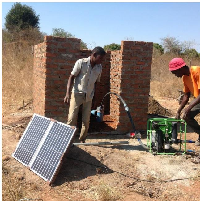
Figure 1 Solar water pump, Source: Celfre
